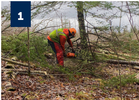
▲ Initial surveying, right-of-way clearing and access routes
