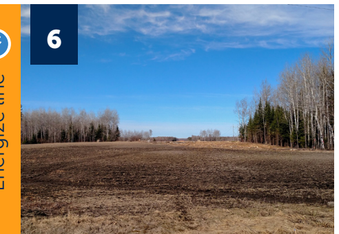
▲ Cleanup and restoration
