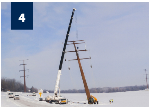
▲ Assemble and set structures
