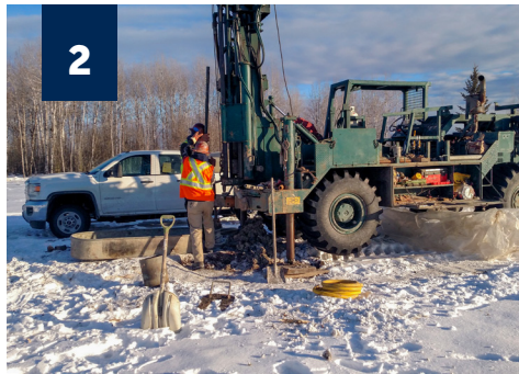
▲ Structure staking, surveying and soils investigations as needed
