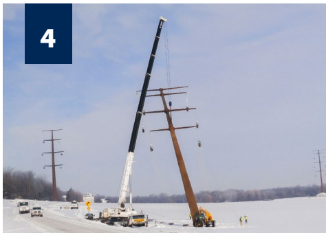
▲ Assemble and set structures
