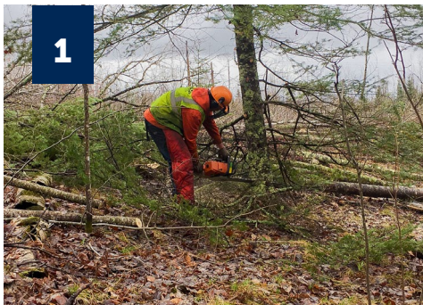
▲ Initial surveying, right-of-way clearing and access routes
