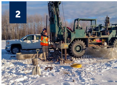
▲ Structure staking, surveying and soils investigations as needed
