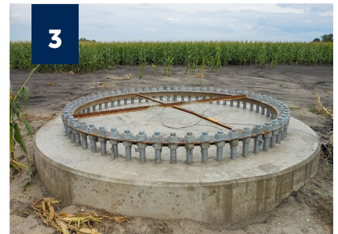
▲ Foundation installation Foundation type may vary depending on structure
